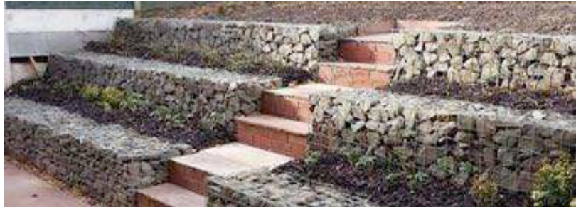
Gabions used as soil retainer on a sloping soil surface
