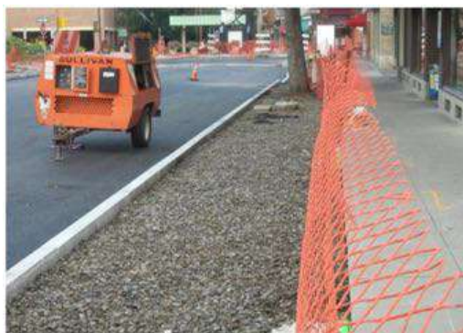
Structural soil (Bassuk et al., 2015)
