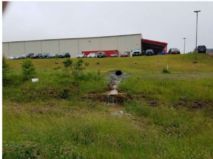
Figure 28: A vegetated water storm basin: a combination of a NBS and a conventional solution
