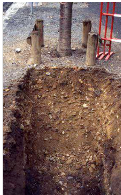
Structural soil profile (© Rossignol)
