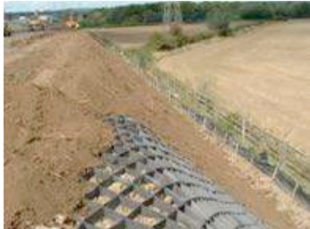
A slope covered with geocell and infilled with topsoil © Terram geosynthetics
