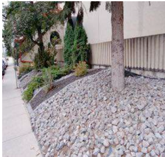
Rock mulch used as soil retainer
