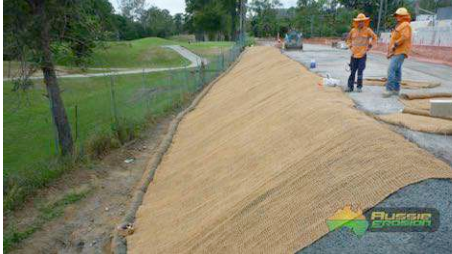
Placement of an coir mesh © Aussie Erosion
