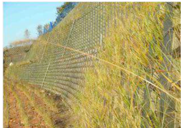
Geocell wall combined with a fiber mat on the same slope surface © Furbish
