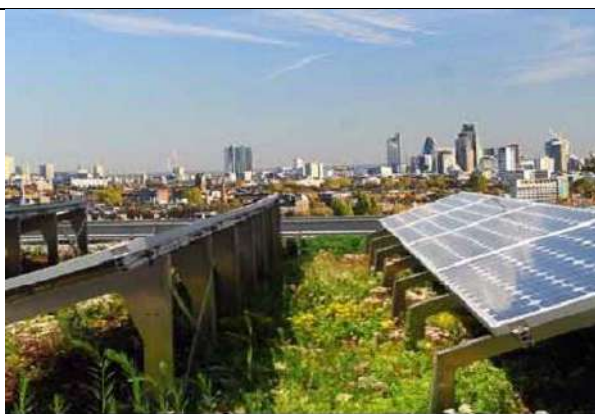
The combination of a green roof and solar panels Photo: Green roofers
