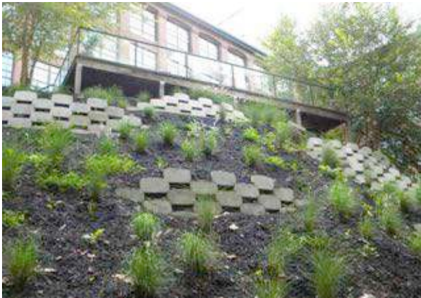
Mulch technics combined with concrete blocks on the same slope surface © Furbish
