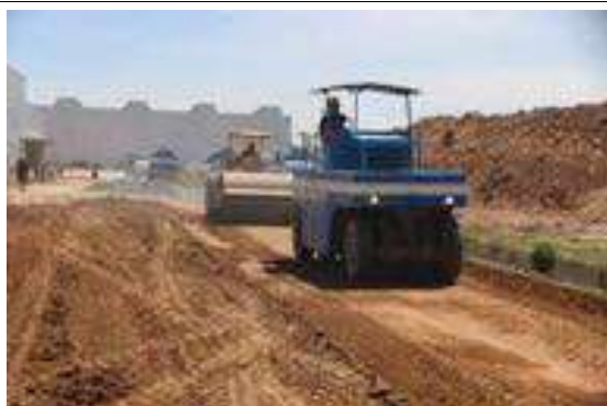
Rolling compaction © Fujiroad
